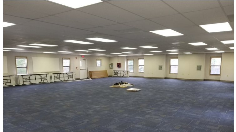
New temporary Dining Hall facility at Skyview
